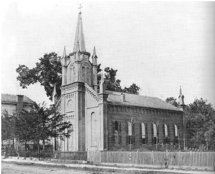
Emmanuel Episcopal Church early 1900s showing Jacob Holt's remodeling. Note the frame siding and lack of stain-glass windows.
